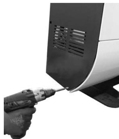
**Fig. 33 - Panel lower fixing**
