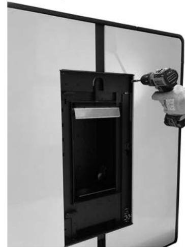
**Fig. 41 - Coating fixing**
