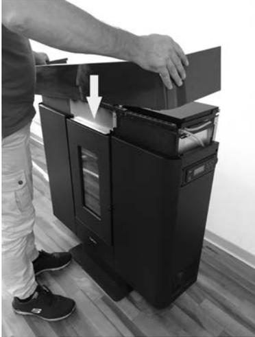
**Fig. 34 - Slide the panel on**
