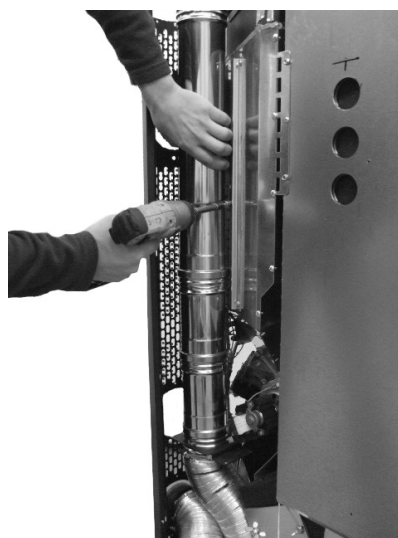
Fig. 63 - Pipe fastening
